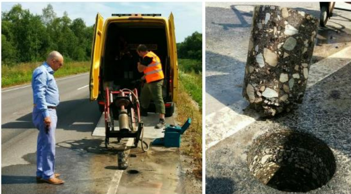
Picture 2. Core drilling of samples for compression strength measurements in N-M.
