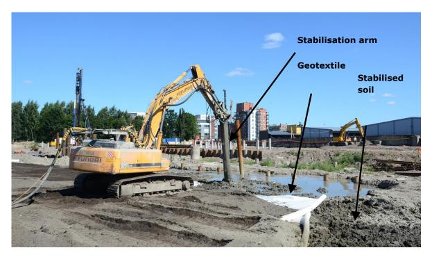
Figure 4-1 Mass stabilisation equipment stabilising clay
