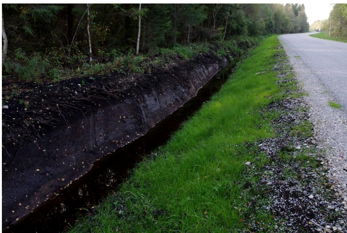
Figure 16. The vegetation in the right (western side) road edge of the middle side of the test section in 2014, view looking to the north. Grass is sown on the road embankment, the dredged outside area is not vegetated (2014, R. Pajula) / Katselõigu keskosa parema (läänepoolse) teeserva taimkate 2014. aastal, vaade põhja suunas. Mulde nõlvale on külvatud muru (2014, R. Pajula)
