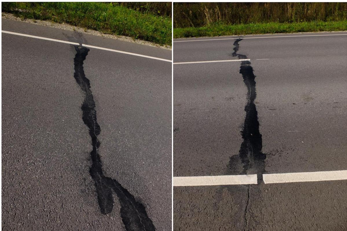
**Figure 6-2. Transverse crack in 2013**
