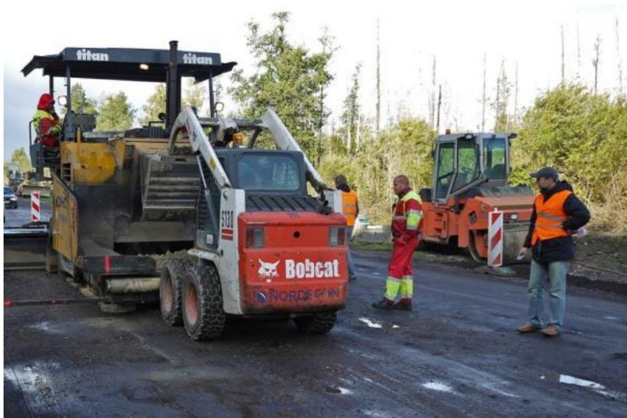
**Figure 4-5. Bobcat filling the asphalt paver punker**
