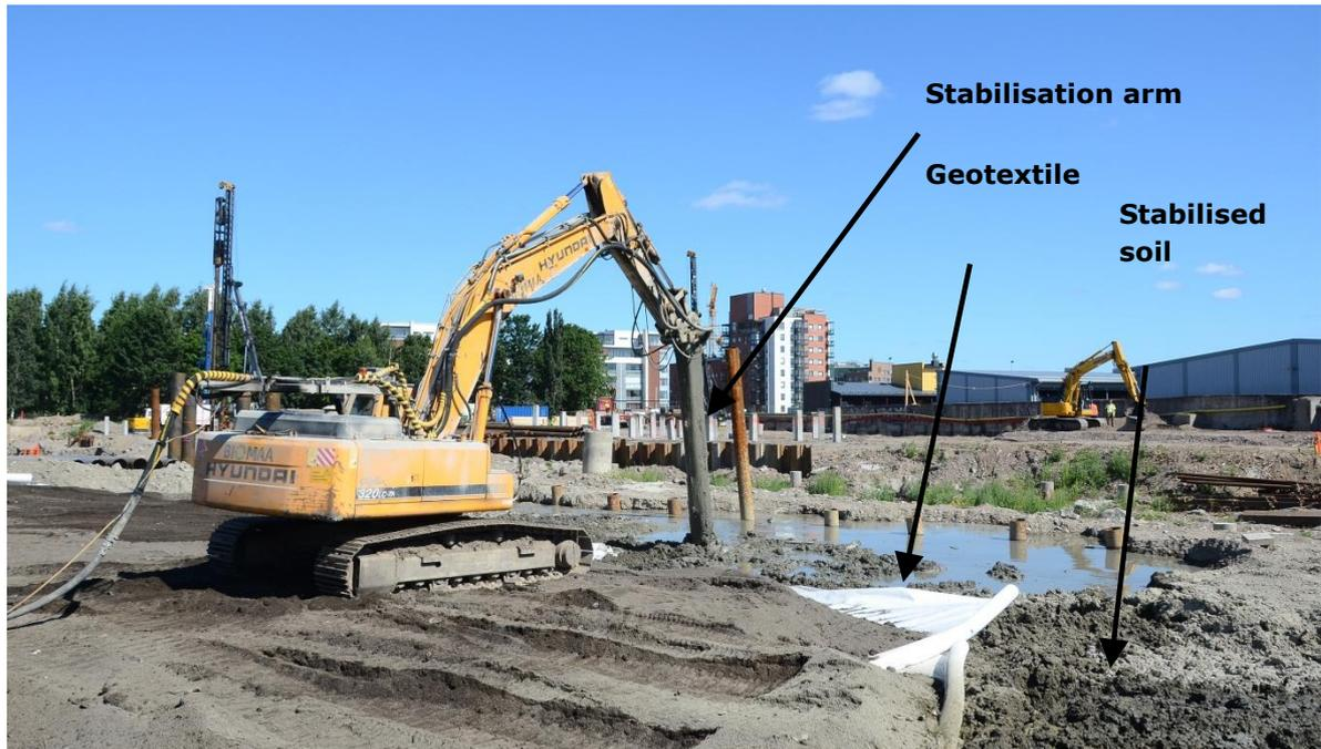
**Figure 4-1 Mass stabilisation equipment stabilising clay**
