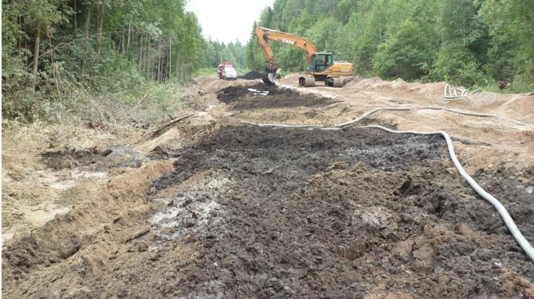
**Photo 4-1 Removal of topsoil**
