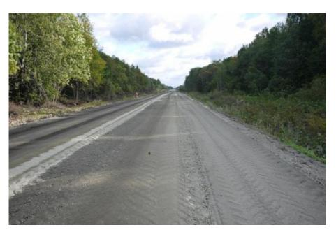
Figure 4-13. Grain size sorting on the surface of freshly stabilised section. The lane was stabilised in two rotary mixer runs and the coarser looking tracks are located in the extreme left side of the Rotary mixer track
