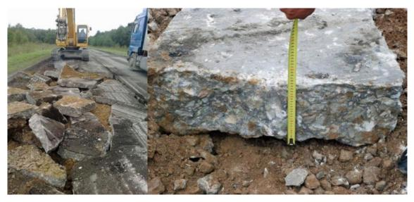
Figure 2-2. The concrete layer found below the pavement
