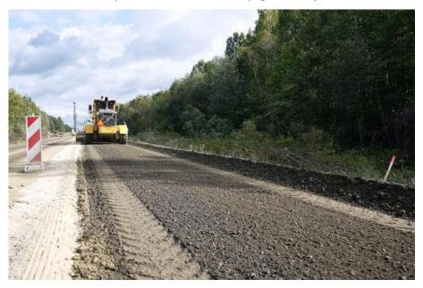
Figure 4-12. Too wet material in the centre sector of freshly stabilised section at STA 8+50
