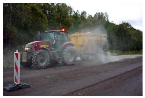
Figure 4-9. Tractor-pulled cement spreading car
