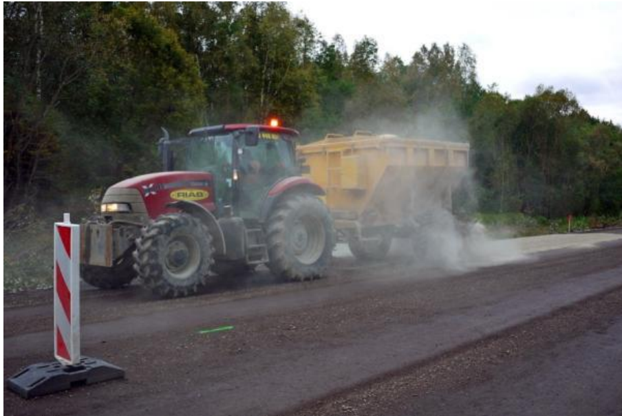
Photo 3-1 Tractor-pulled cement spreading device
