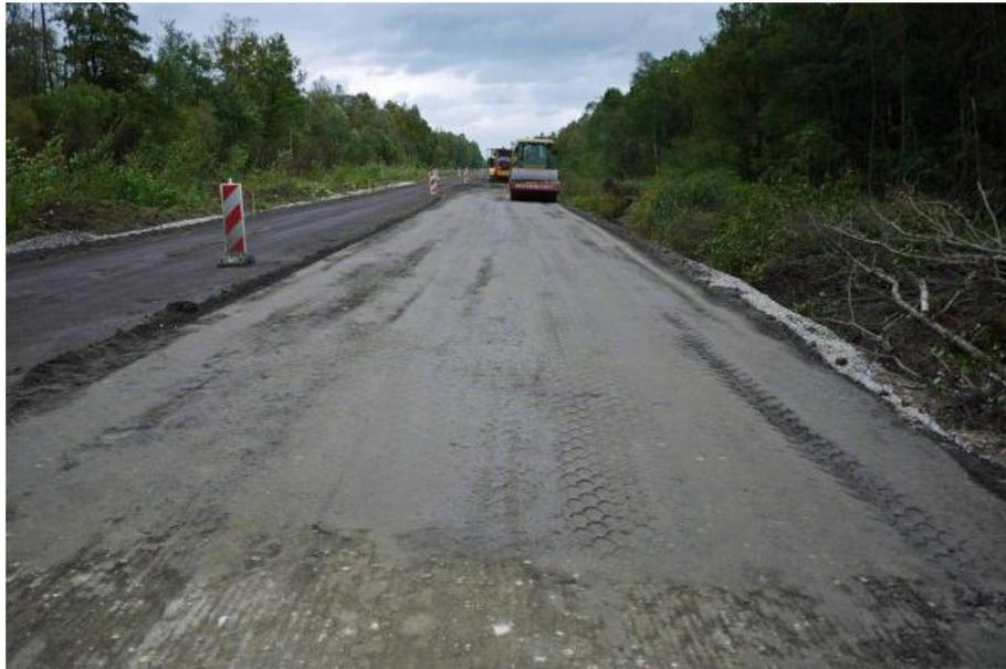
**Figure 4-8. The first batch of stabilisation mixing after grading and compaction**
