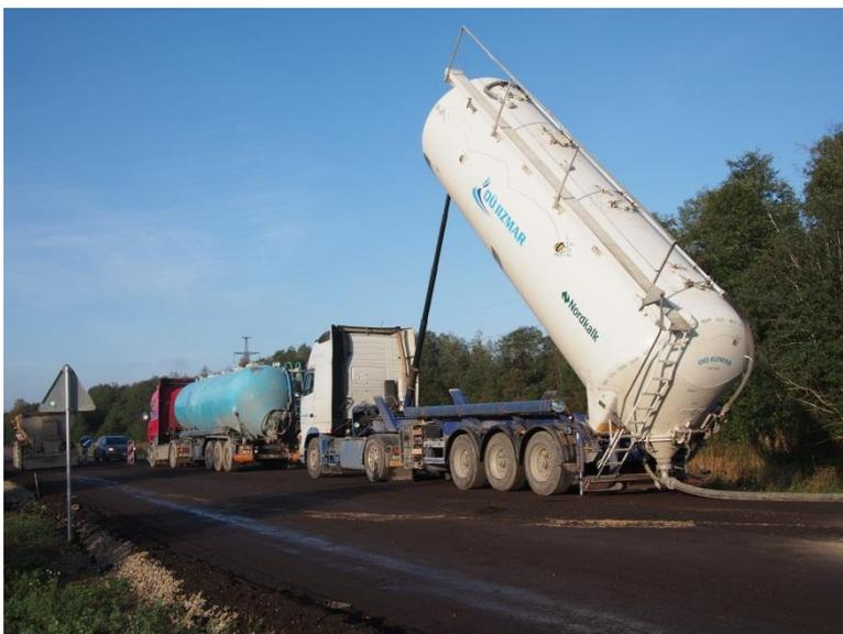
**Figure 4-14. Binder transporting to the construction site**
