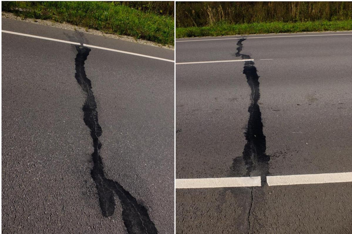
**Figure 6-2. Transverse crack in 2013**
