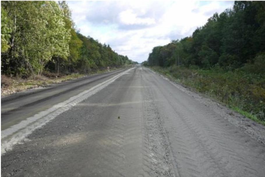
**Figure 4-13. Grain size sorting on the surface of freshly stabilised section. The lane was stabilised in two rotary mixer runs and the coarser looking tracks are located in the extreme left side of the Rotary mixer track**
