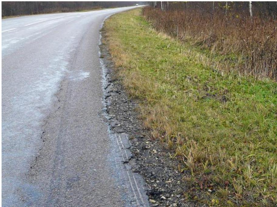
**Figure 3-10. AC surface set lower on road side (Oct 2010)**
