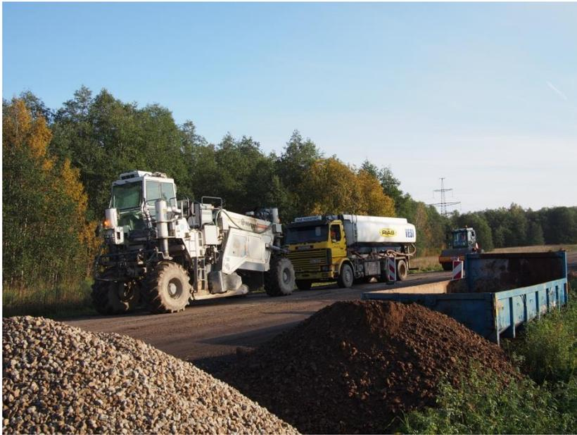
**Figure 4-15. Rotary mixer and water transporting**
