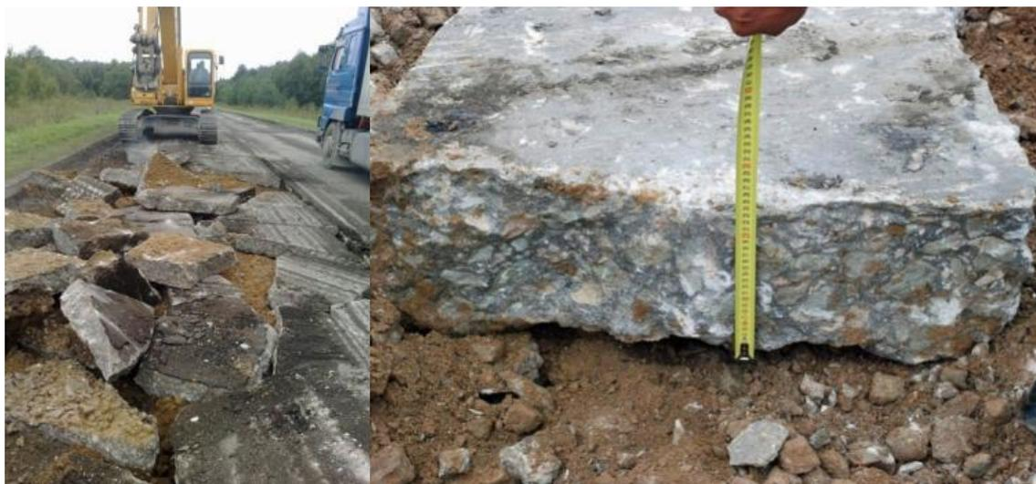
**Figure 2-2. The concrete layer found below the pavement**
